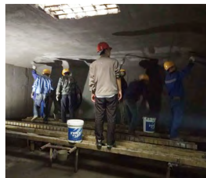
Almost 10,000 square meters of crack sealing and durability enhancing Xypex Concentrate treatment were applied at the direction of engineers of the Chishi Bridge recovery team.
