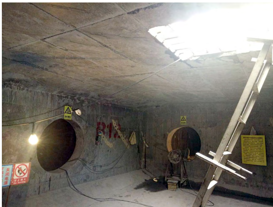
Almost 10,000 square meters of crack sealing and durability enhancing Xypex Concentrate treatment were applied at the direction of engineers of the Chishi Bridge recovery team.
